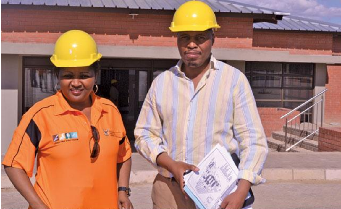
Delivering healthcare infrastructure ... Public Works MEC, Sisi Mabe, inspecting the construction site of Matsopa Hospital
